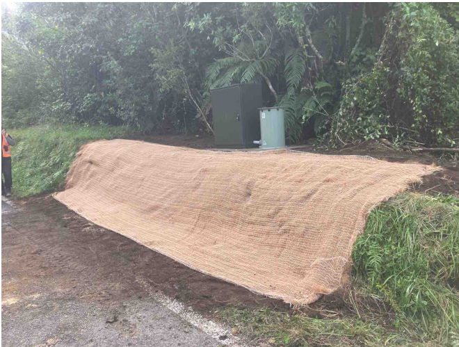
Completed Air Valve and Odour Filter Installation
