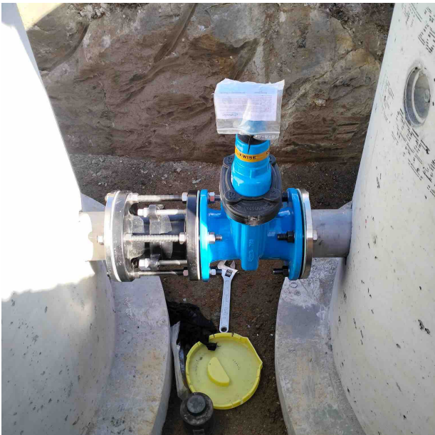
Cliff Road Pump Station – Isolation valve installation
