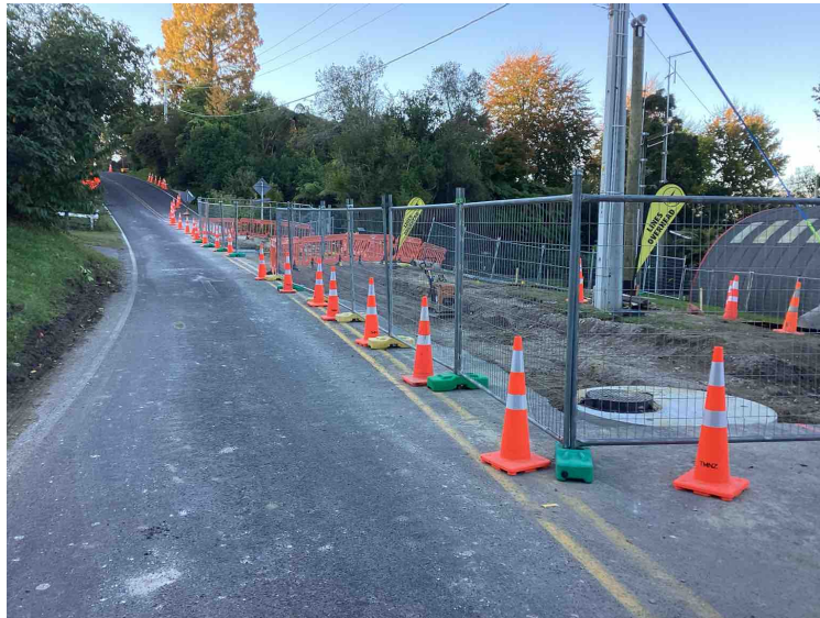
Stoney Point Pump Station – Storm water diversion works
