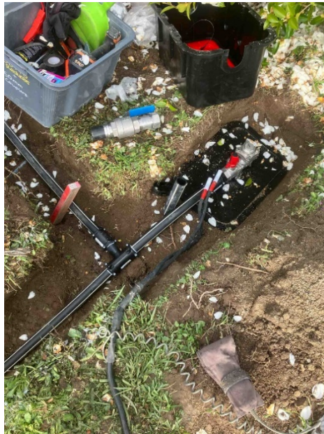
Boundary Assembly installation
