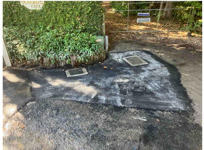
Asphalt reinstatement at the end of Ronald Road
