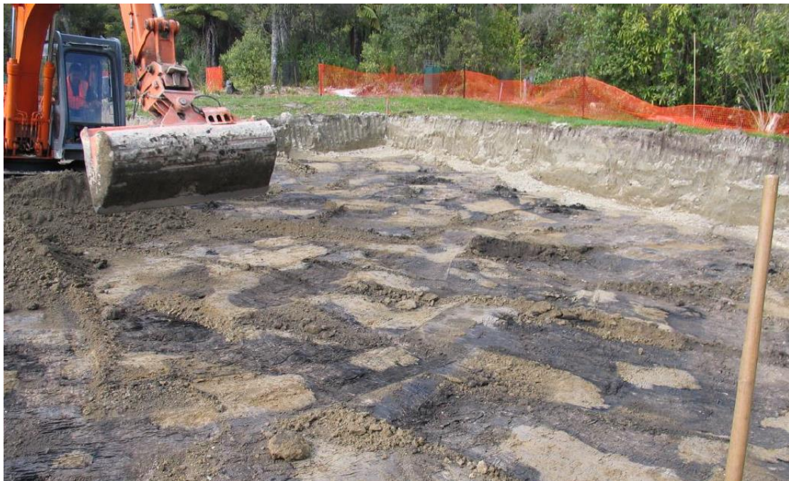
Figure 14. Photo showing 1m deep Rotomahana mud covering the pre 1886 topsoil within 7 Rangiuru Bay Road. Phillips 2015a.
