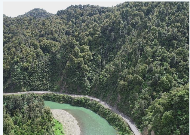
(A) Deeply incised Waioeka Gorge, with active and recent instability on the steep natural hillslopes and road cuts
