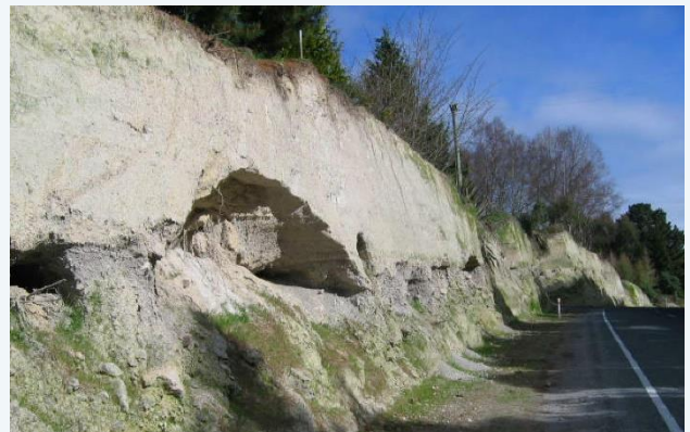
(B) Loose tephra (pumice and ash deposits) exposed in road cutting
