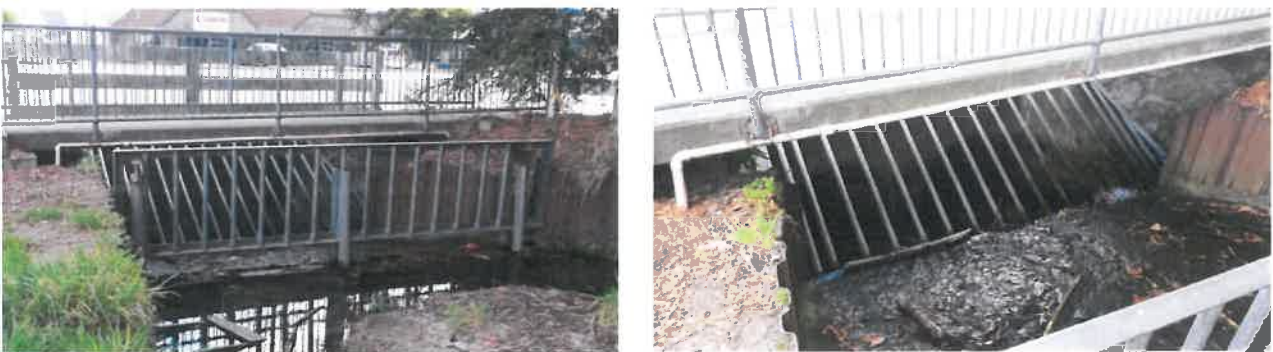
Figure 3-5: Inlet to Te Ngae Road screened culvert
