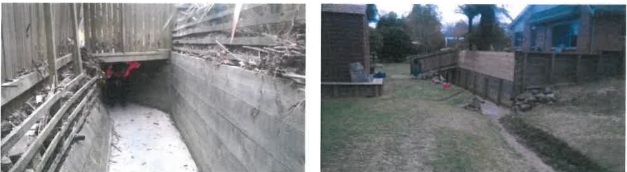
Figure 3-3: Selwyn-Larcy drain final wooden section (left) and poorly formed channel upstream of wooden section (right)
