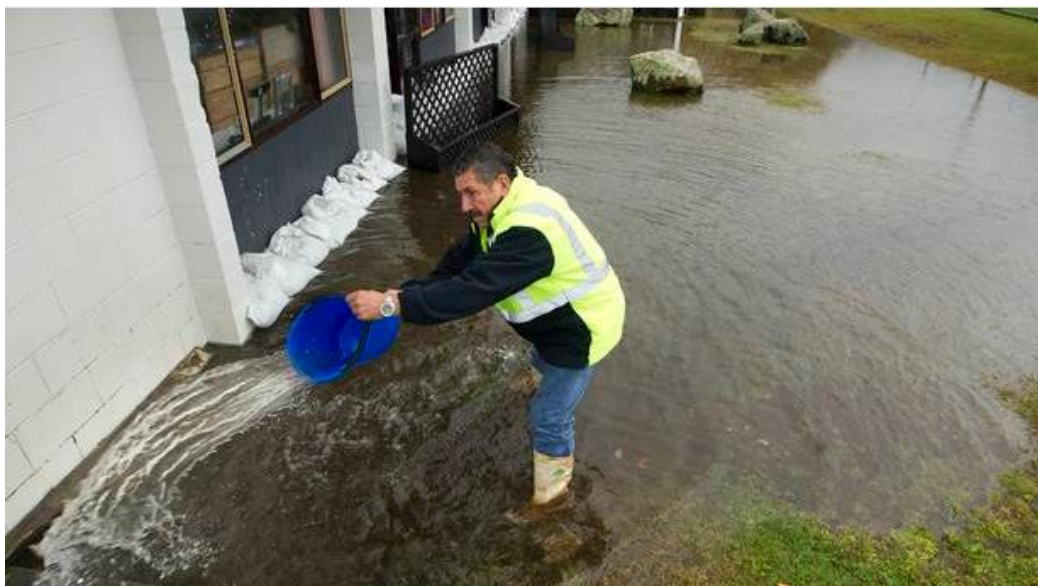
Figure 11: Rotorua Daily Post photo - Flooding at Waikite Rugby Club April 2018
