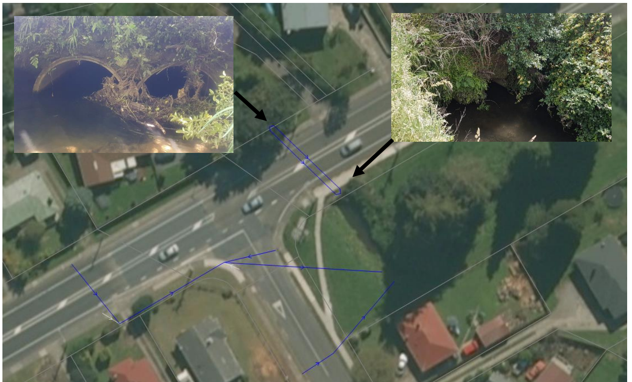
Sunset Road Culvert
