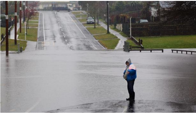
Figure 4-4: Flooding at Ford Road (taken looking north towards the Ford Road culvert)
