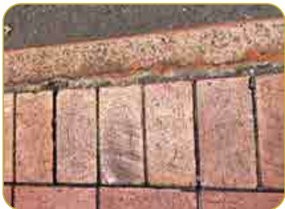
Figure 16 Concrete edging at ground level affected by geothermal conditions (photo: Kim Smith, January 2024).
