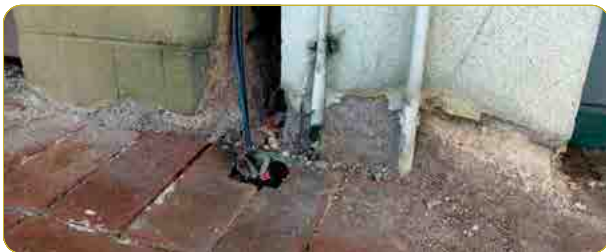
Figure 24 Deterioration of building materials at ground level (photo: Kim Smith, January 2024).
