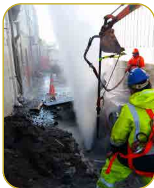
Figure 4 Bore Failure, 2016 (photo: Andrew Austin).
