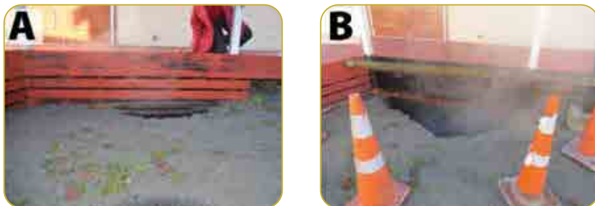
Figure 10 A collapse hole developing at Whakarewarewa Village over eight days in September 2012. Roof-fed stormwater disposal to shallow depth drove the creation of the feature (these images were originally published in Fitzgerald, 2022)
