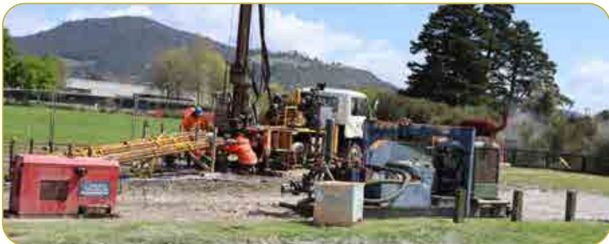
Figure 22 Example of space required around a bore for a drilling rig and plant (photo: Rotorua Well Drillers).
