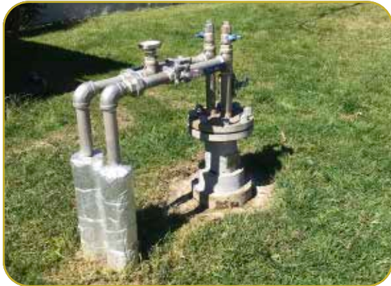
Figure 13 Bore examples. To the left is a typical heat exchange bore. In the example to the right the lower part of a gas vent can be seen at the top of the well (photos: Rotorua Well Drillers)
