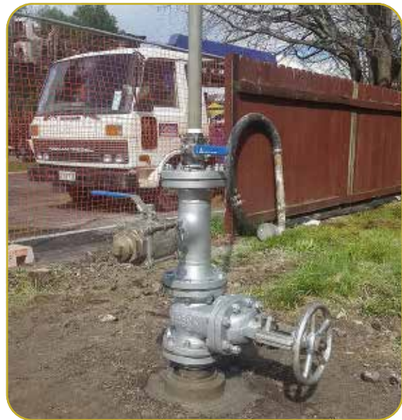
Figure 13 Bore examples. To the left is a typical heat exchange bore. In the example to the right the lower part of a gas vent can be seen at the top of the well (photos: Rotorua Well Drillers)
