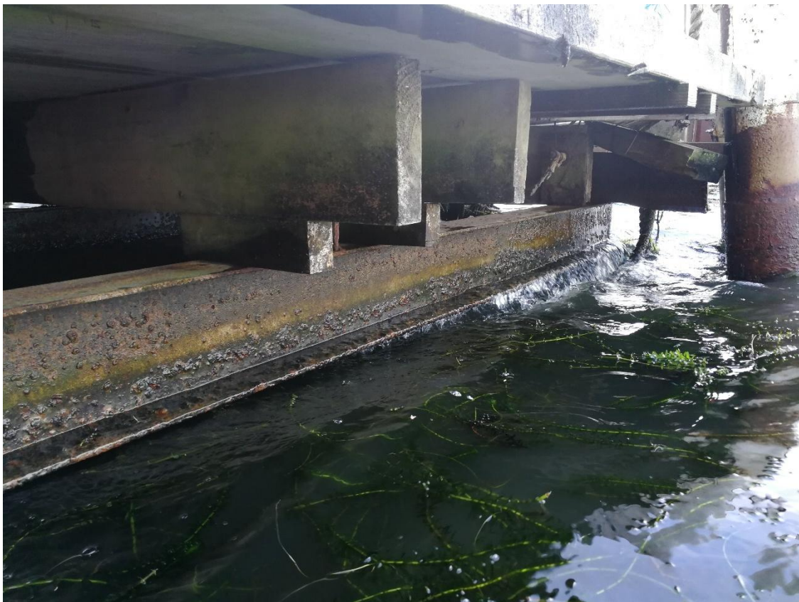
Photograph Appendix A.4: Lakeland Queen Wharf Head support structure- 2
