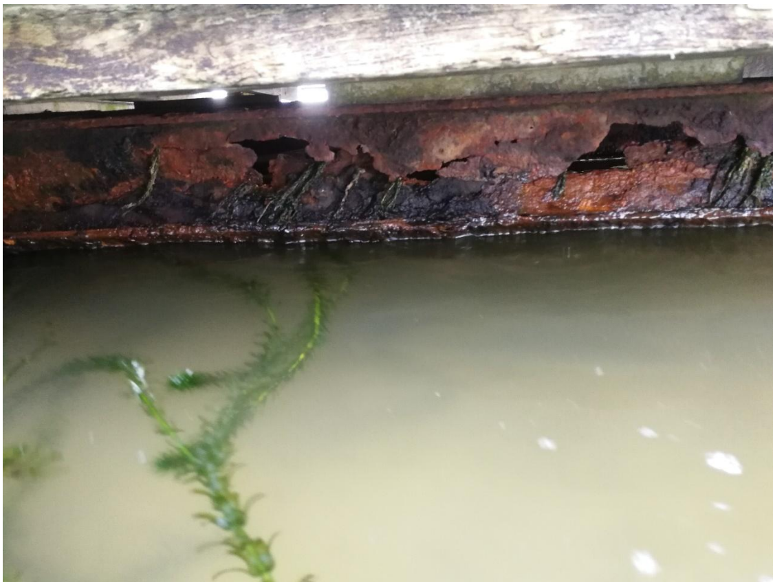
Photograph Appendix A.10: Lakeland Queen Wharf Head 200 UB edge beam
