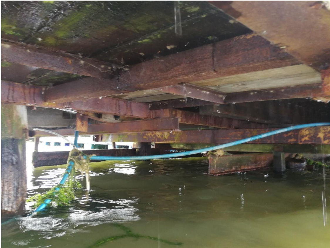
Photograph Appendix A.3: Lakeland Queen Wharf Head support structure- 1
