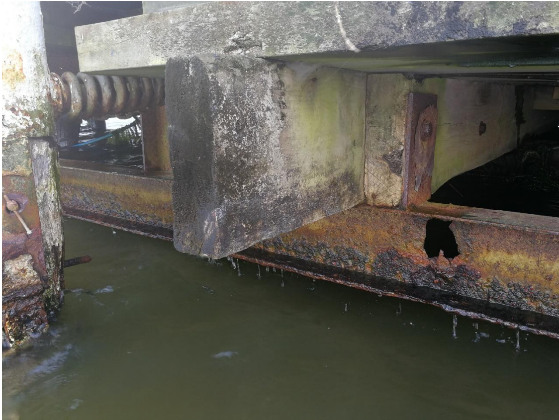
Photograph Appendix A.9: Lakeland Queen Wharf Head 200 UB edge beam
