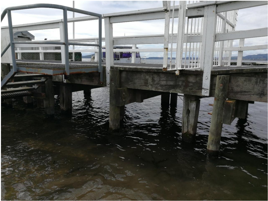
Photograph Appendix A.13: RLC Wharf - general
