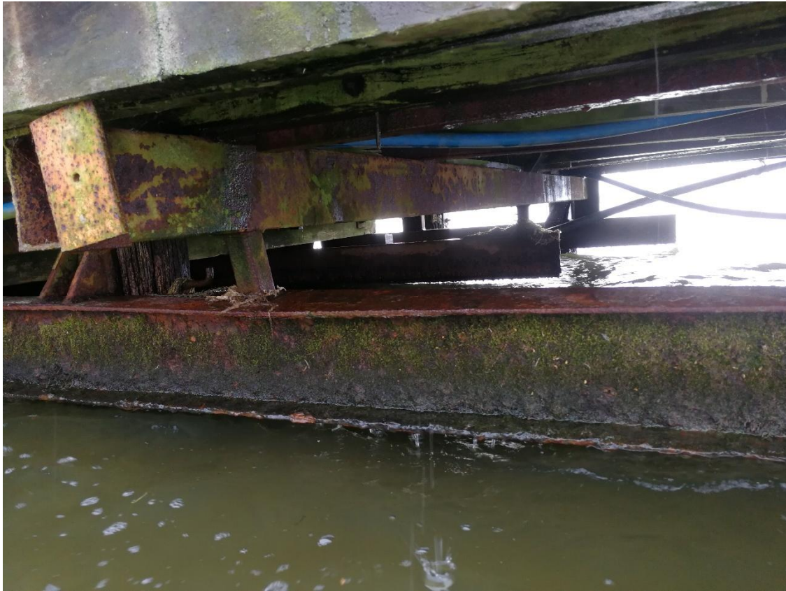
Photograph Appendix A.11: Lakeland Queen Wharf Head support structure
