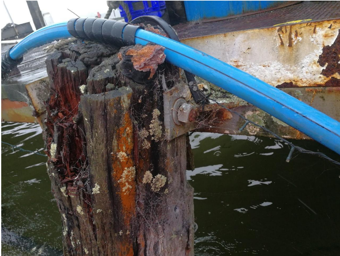
Photograph Appendix A.7: Lakeland Queen Wharf Head pile - 1
