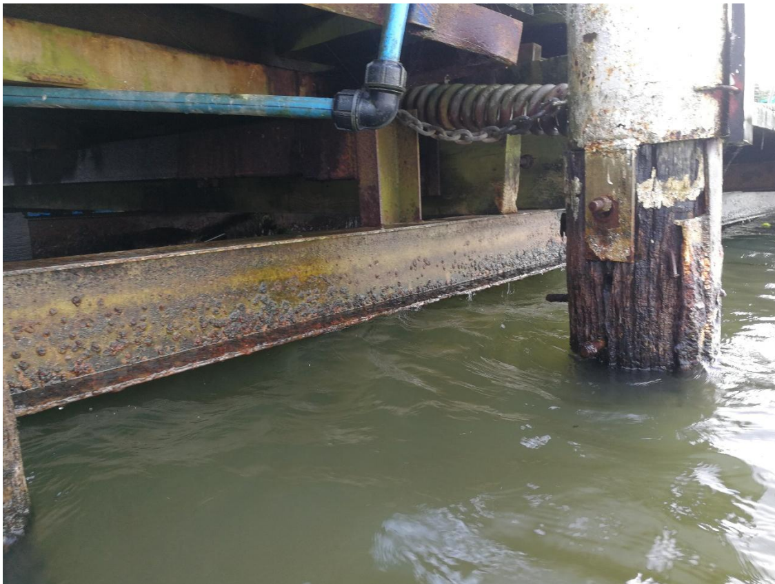
Photograph Appendix A.6: Lakeland Queen Mooring Pile
