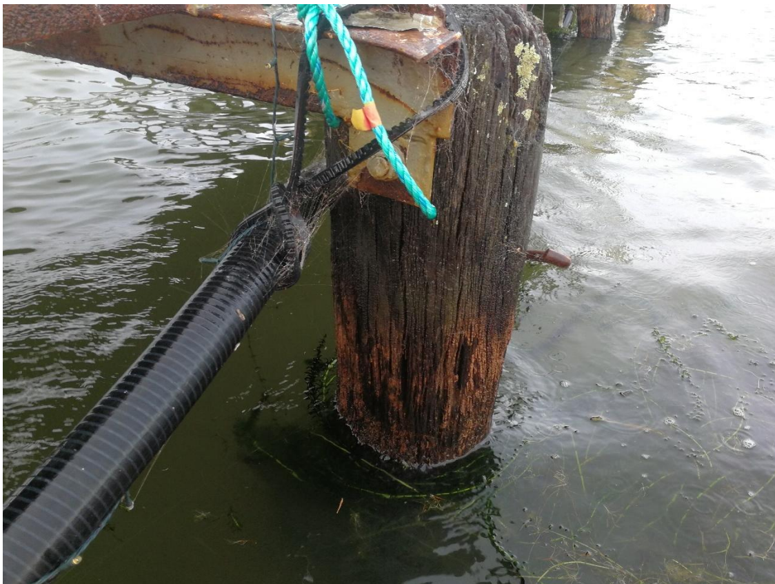
Photograph Appendix A.8: Lakeland Queen Wharf Head pile - 2
