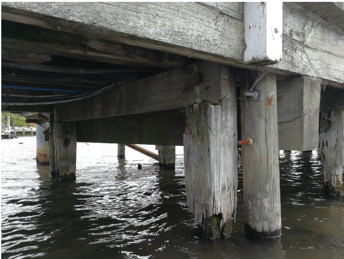
Photograph Appendix A.12: RLC wharf – piles and bearer
