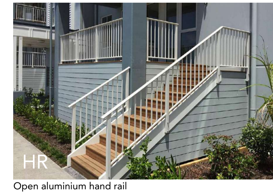
HR Open aluminium hand rail
