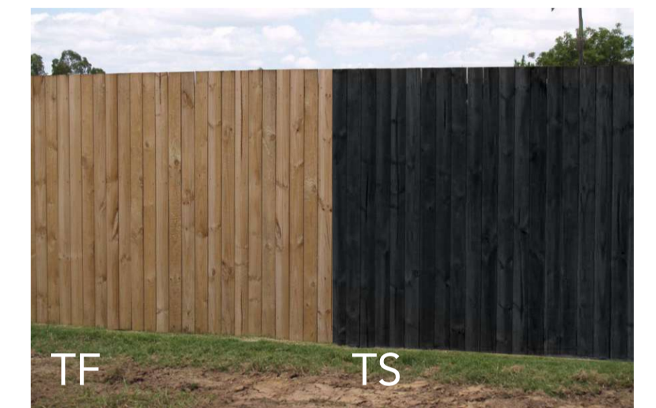
TF 1.8m Timber paling fence
