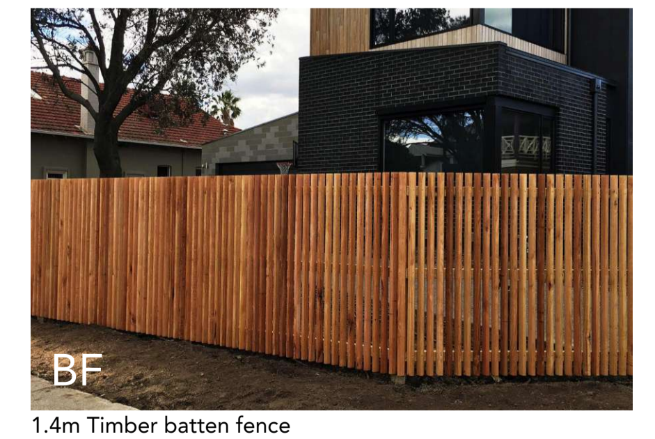
BF 1.4m Timber batten fence
