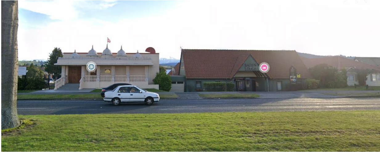
Figure 3: 303 Fenton Street (Shri Swaminarayan Mandir Temple) and 301 Fenton Street (Baden Lodge) (source: Google Street View)
