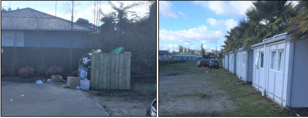
Image 1 & 2: Waste Management area and rubbish outside units.
