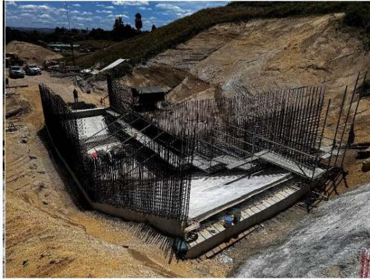
Western Dam auxiliary spillway construction
