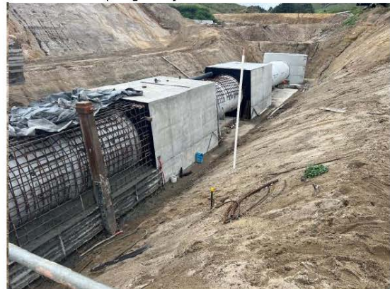
Eastern Dam - construction of the primary spillway
