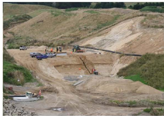
Eastern Dam progress from above
