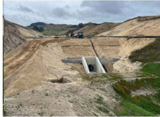
Eastern Dam progressing above the ground
