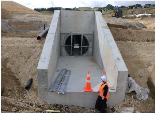
Western Dam - construction of the primary outlet
