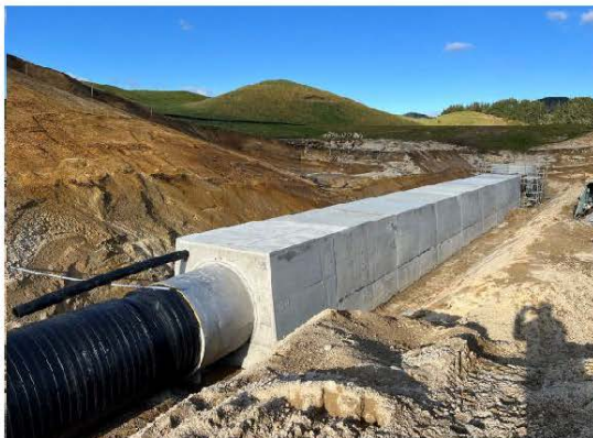
Western Dam - construction of the primary spillway
