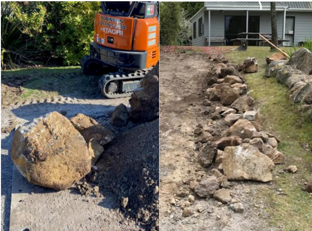
Rocks Encountered during Boundary Connection Install
