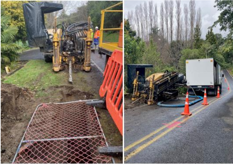
Directional Drilling Equipment Setup
