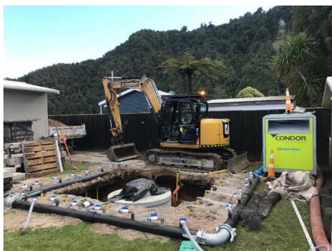
During and after installation - aggregate hardstand area constructed around trafficable system along with additional drainage requirements in front of garage.
