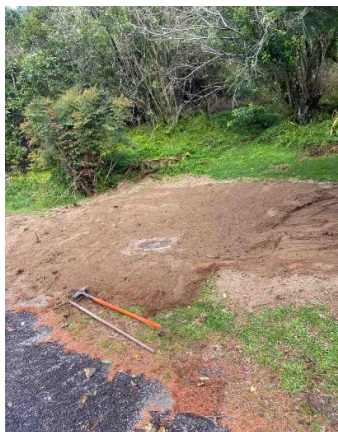
Preliminary reinstatement around a newly installed fibre communications
