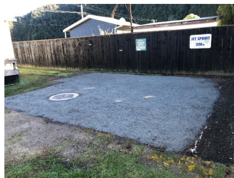
During and after installation - aggregate hardstand area constructed around trafficable system along with additional drainage requirements in front of garage.
