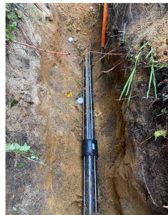
Electrofusion coupler welded in place to join the directional drilled
