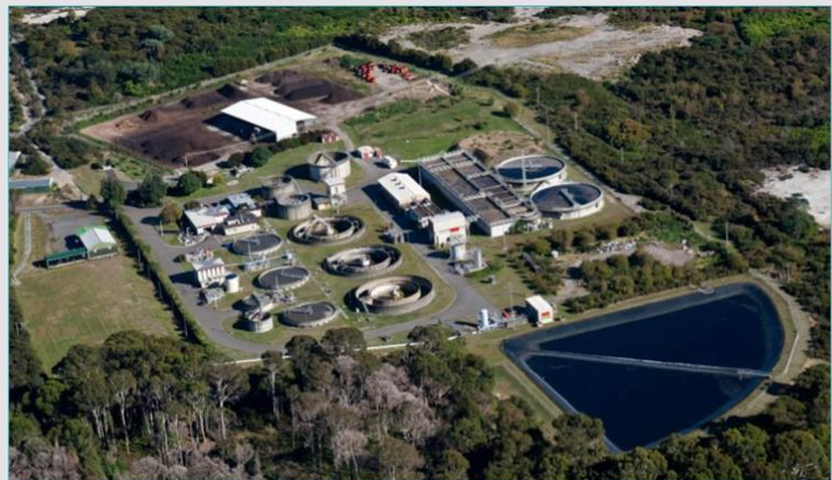
Rotorua Wastewater Treatment Plant now
