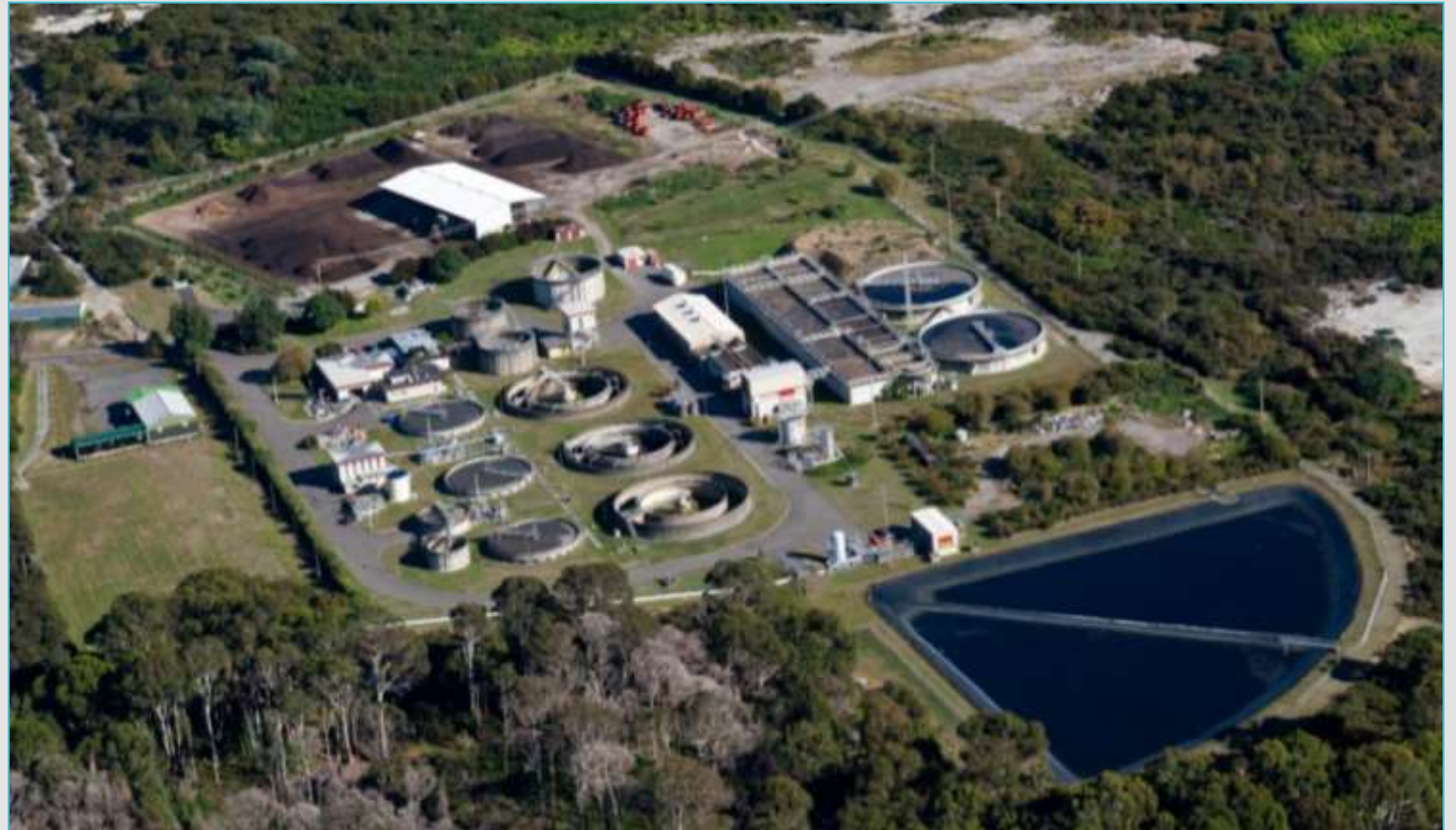
Rotorua Wastewater Treatment Plant now
