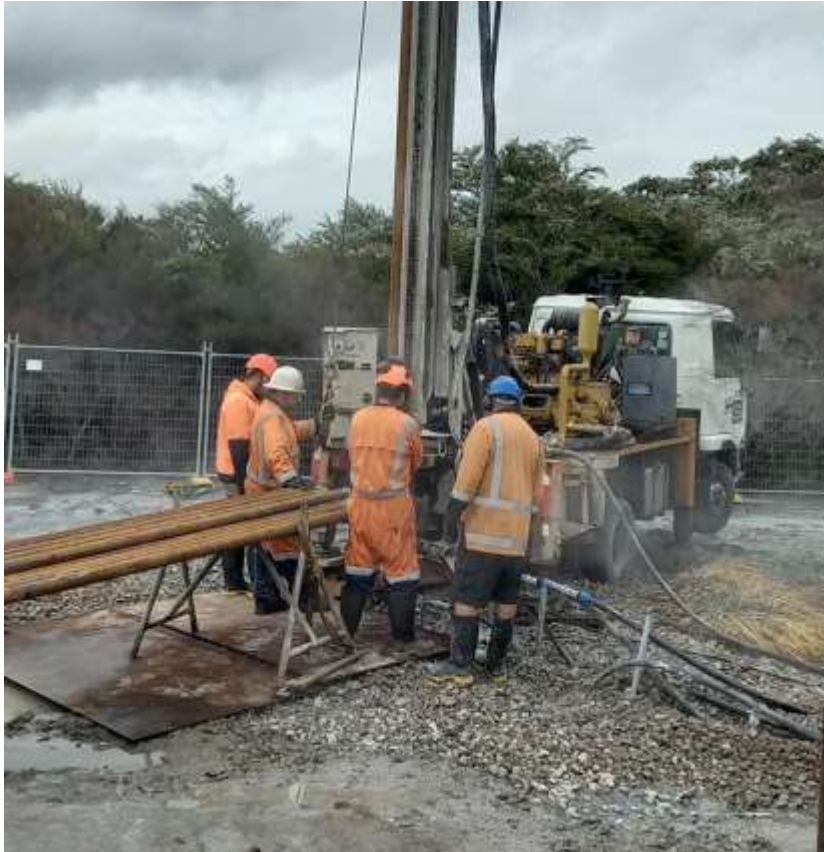
Above: Well drilling crews hard at work in behind the EEC
