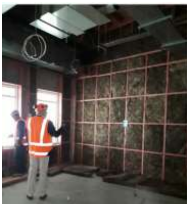
First floor studio north wing sound proofing and HIVAC installations
