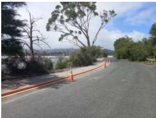
Above: Kerb and channel along Hatupatu Drive for new cycleway edging
