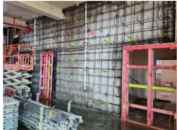
Additional sheer was waiting for concrete for concrete pour as part of strengthening
