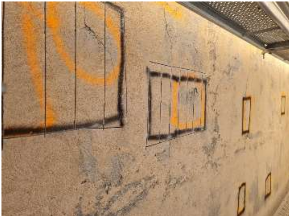
Drummy plaster identified to be removed and replaced
