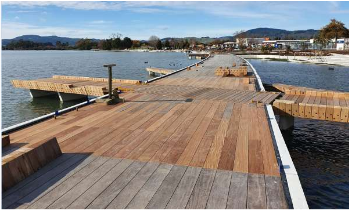
Stage 1 Boardwalk and Tukutuku bridges nearing completion
