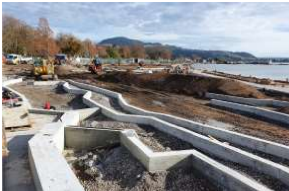
Stage 1 Eastern end terraces and landscaping
