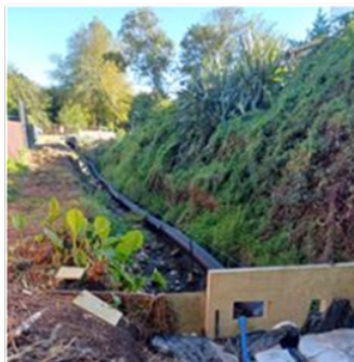
Pictured: Pipe diversion and temporary dam for planned works
