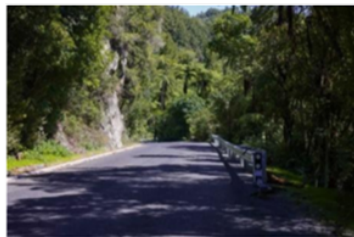
Widening of road
