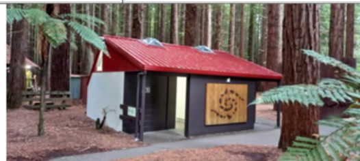
Newly refurbished toilets at the Redwoods I-site
