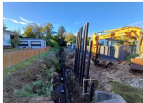
Pictured: Installation of pilings to stabilise drainage bank
