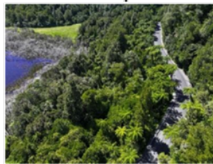
Aerial image of completed work
