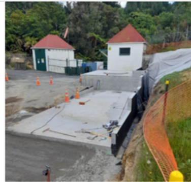
Pictured: Central delivery bund and storage tank foundations
