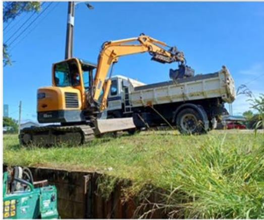
Above: Melrose Avenue major clearance of timber lined drain
