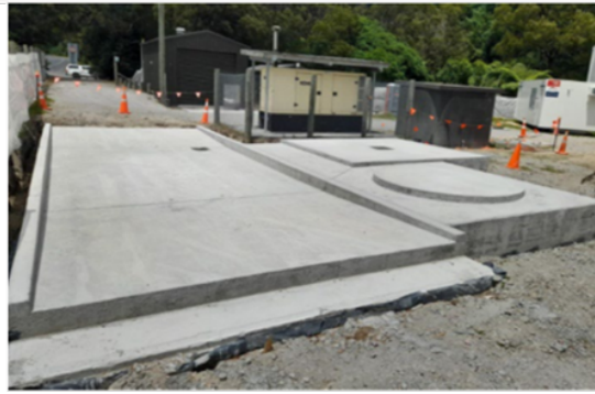
Pictured: Eastern delivery bund, storage tank and building foundations
