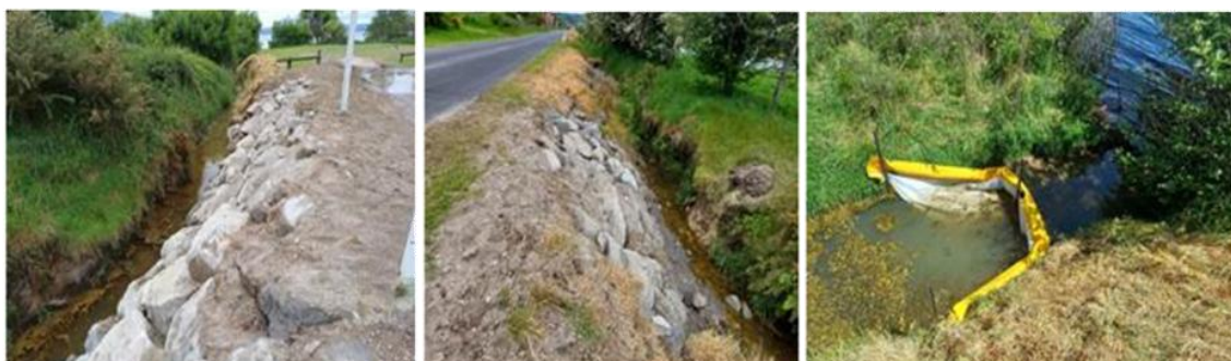
Owhata Road Drain wall repairs
