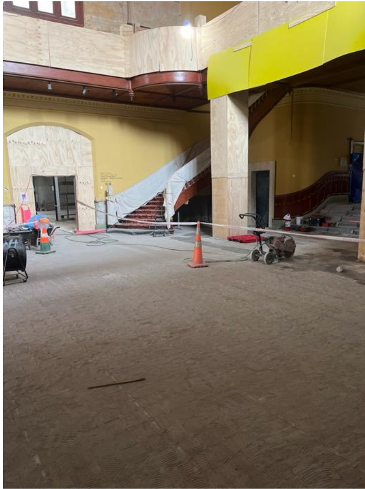
Figure 6: Atrium floor tile removal 11/11
