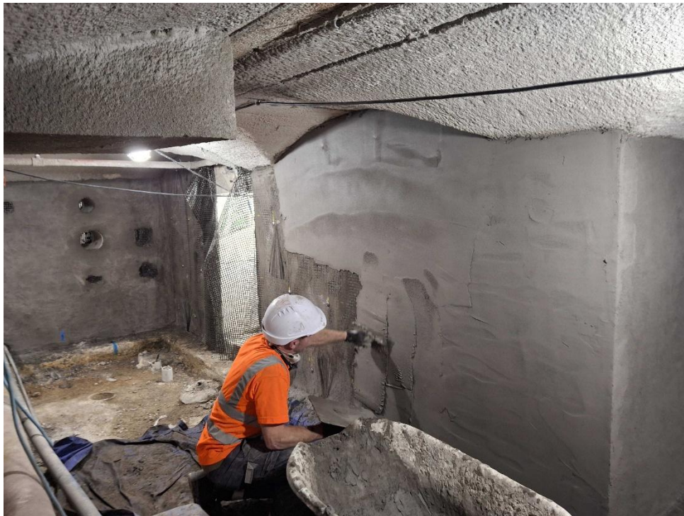
Figure 3: FRM wall application 30/10
