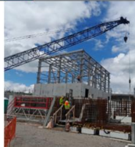
Installing transformer pads for WWTP electrical power supply.
