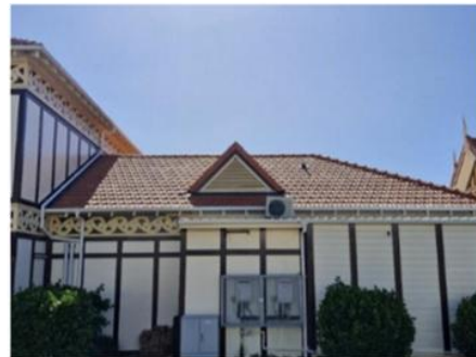
Completed roof replacement
