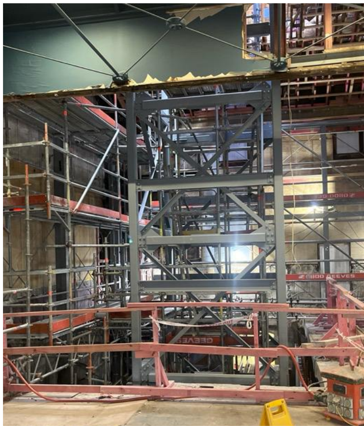
Figure 5: Lift shaft steel erection 11/11
