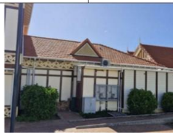
Completed roof replacement at city iSite
