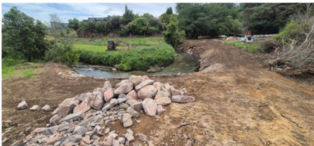
Baxendale Reserve stream edge erosion protection
