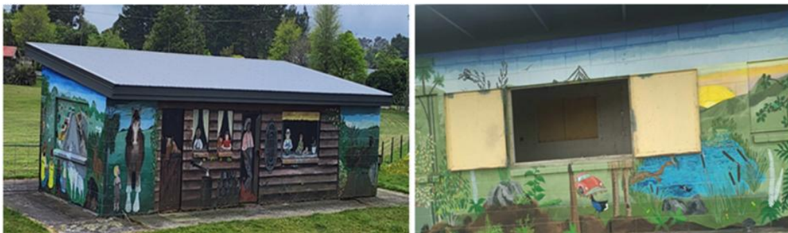
Mamaku Pavilion restored
