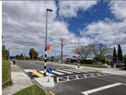
New pedestrian crossing outside Rotorua Lakes High School, Porikapa Road
