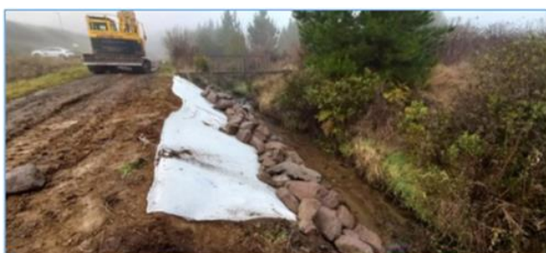
Photo above: Armouring the embankment on the dog pound stream
