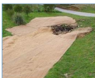
Photos above: Issues with a swale and outfall from a culvert in Redwood Park prompted excavation of the outlet and clearance of the blocked culvert by DDL/Goodricks. Coconut cloth installed for stabilisation of the ground to prevent scour.
