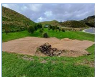
Photos above: Issues with a swale and outfall from a culvert in Redwood Park prompted excavation of the outlet and clearance of the blocked culvert by DDL/Goodricks. Coconut cloth installed for stabilisation of the ground to prevent scour.
