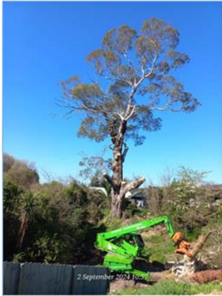
Photo above: Tree Control contractors removing trees from Caufield Place Gully
