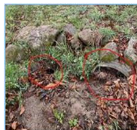
Photos above: Issues with a swale and outfall from a culvert in Redwood Park prompted excavation of the outlet and clearance of the blocked culvert by DDL/Goodricks. Coconut cloth installed for stabilisation of the ground to prevent scour.
