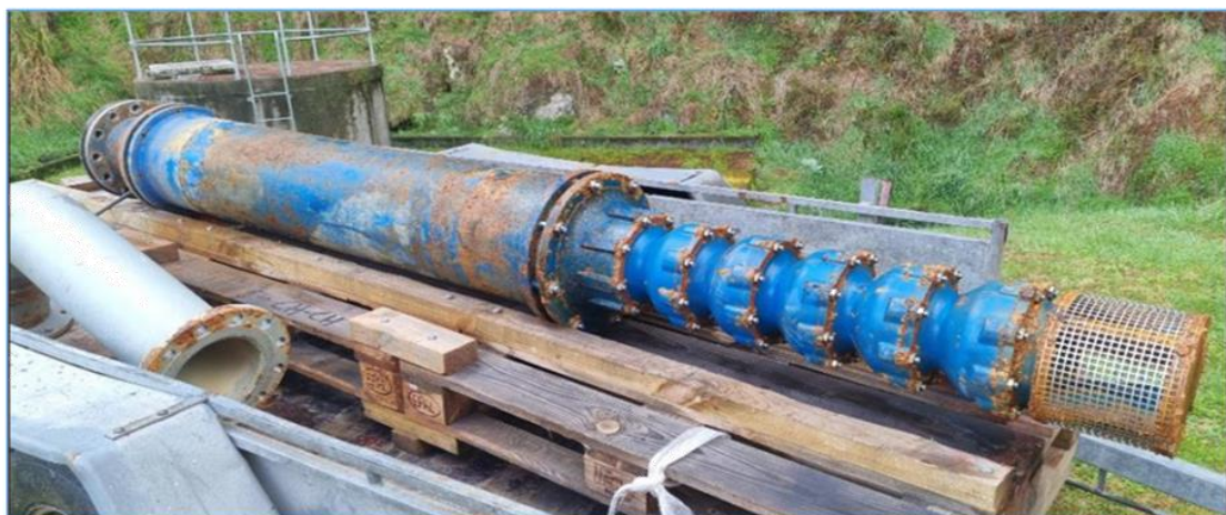
Photo above: The third pump at Deep Creek has been removed for a full service as part of our routine maintenance program. It will be sent to Christchurch to the authorised Plueger agent for New Zealand for full reconditioning to as-new condition.
