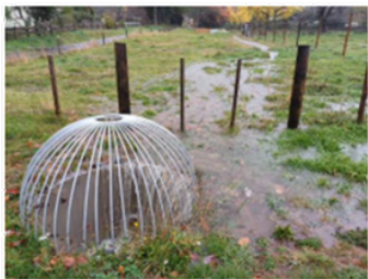
Photo above: Clayton Road scruffy dome is collecting run-off from Mountain Road but further improvements are needed to capture more of the overland flow
