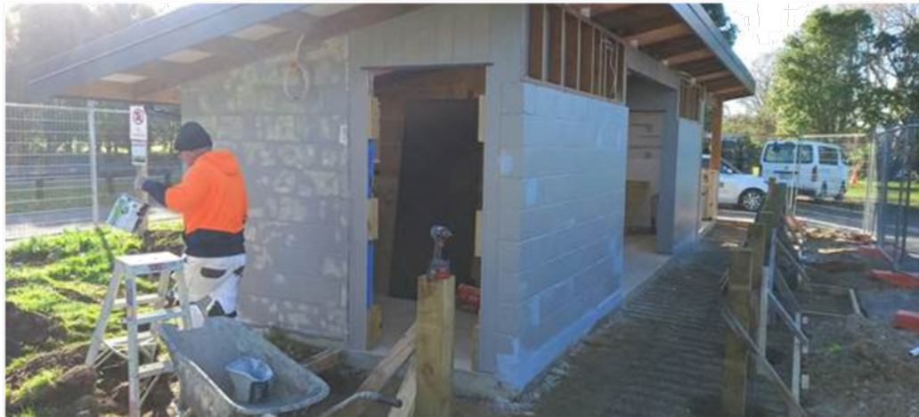
Photo: Eastern Hamurana Toilet block refurbishment underway
