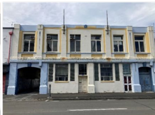
Deteriorating building, Lowe St
