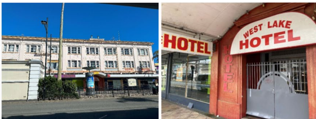
Former Westlake Hotel, Corner Gladstone Rd and Peel St
