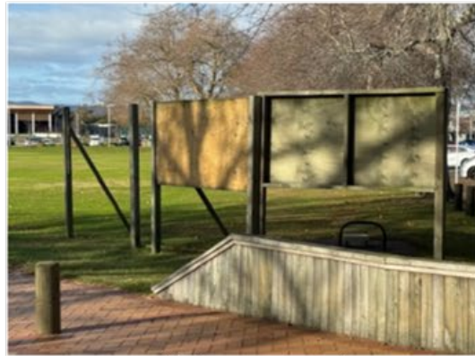
Old signage removed
