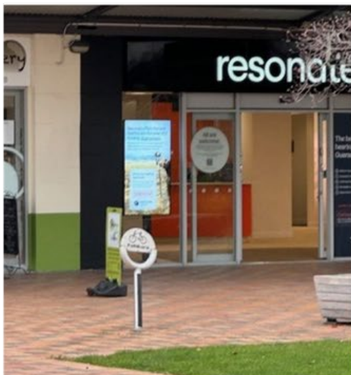
Bicycle stands leaning over and loose
