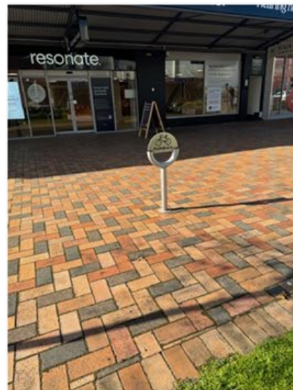
Bicycle stands repaired
