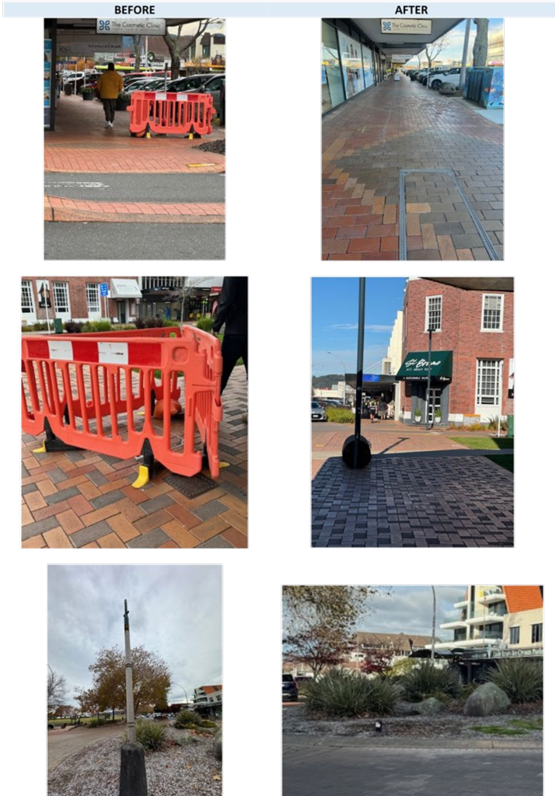
Old broken light post removed
