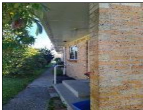
Front entrance in block
