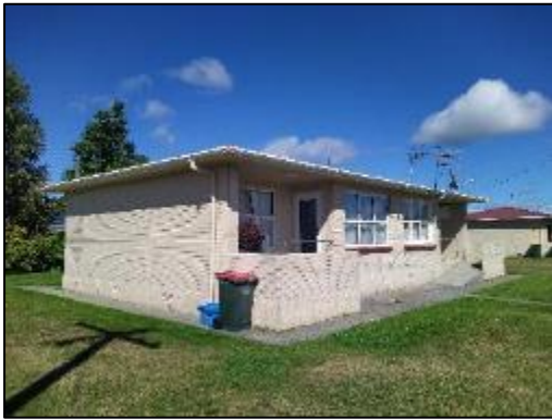
Exterior – Units 53 & 54 in block of 2 attached units
