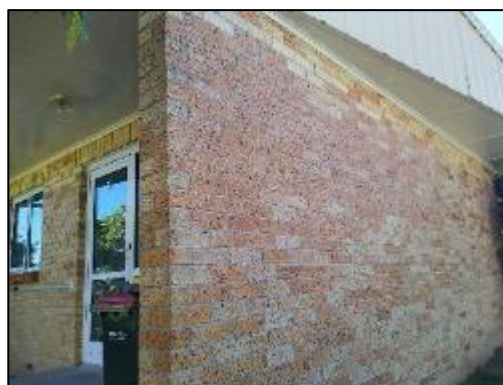
Front entrance, exterior end wall
