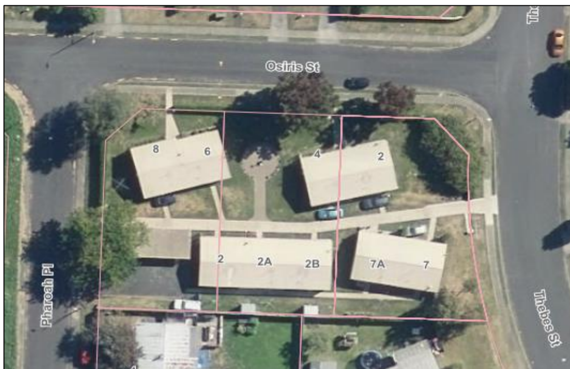
Aerial photo of the 9 Units at the corner of Thebes Street, Osiris Street and Pharoah Place, Rotorua
