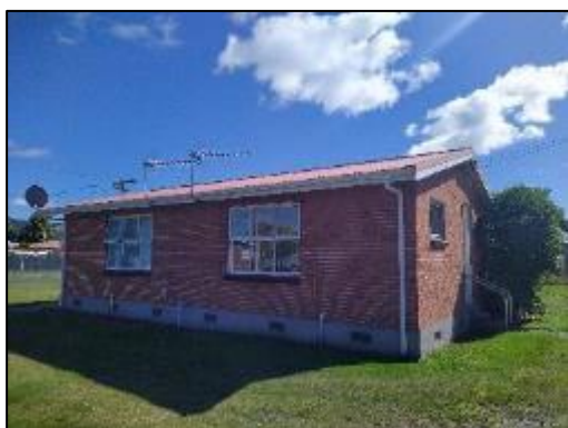
Exterior – Units 37 & 38 in block of 2 attached units
